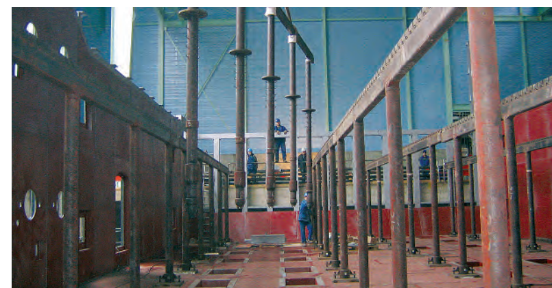
Top: Manufacture of skid pipes for pusher-type furnaces. Bottom: Installation of skid frames at walking beam furnace.
